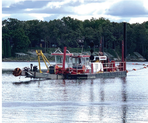
Dredge and floating pipe for removing sediment.
