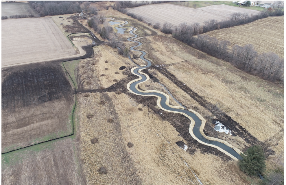
Mason Creek after re-meander completed, November 2022. Re-meandered with tapered banks integrated into floodplain.
